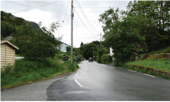
Over. Krohnegården. Fortau mangler (65)
