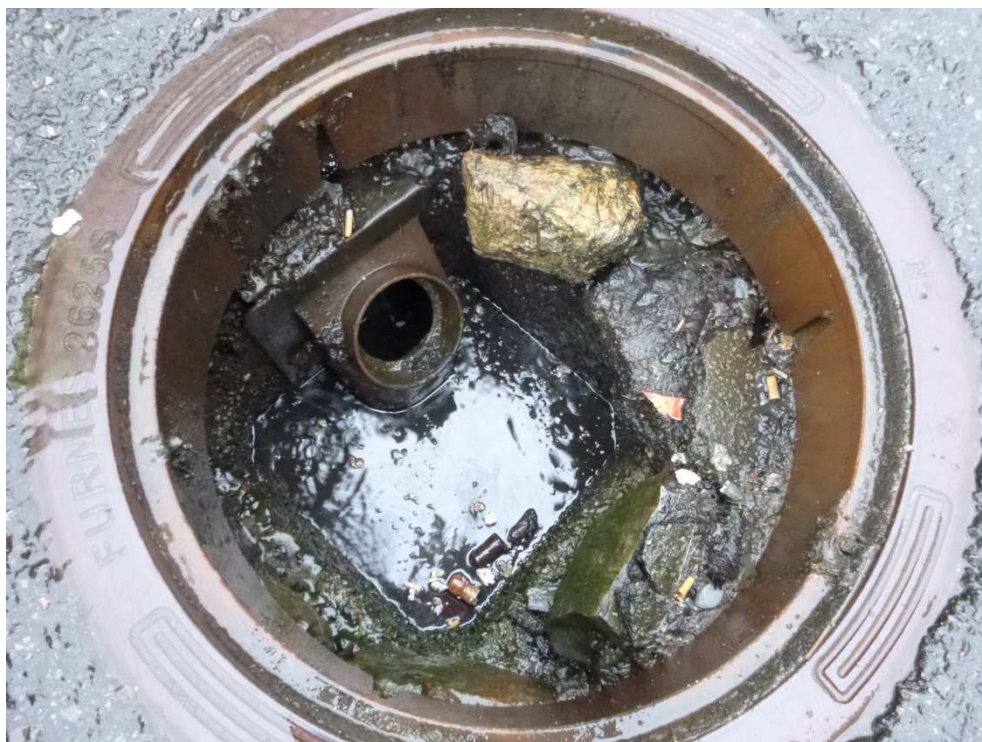
Sandfang 6- C. Sundts gate 55
