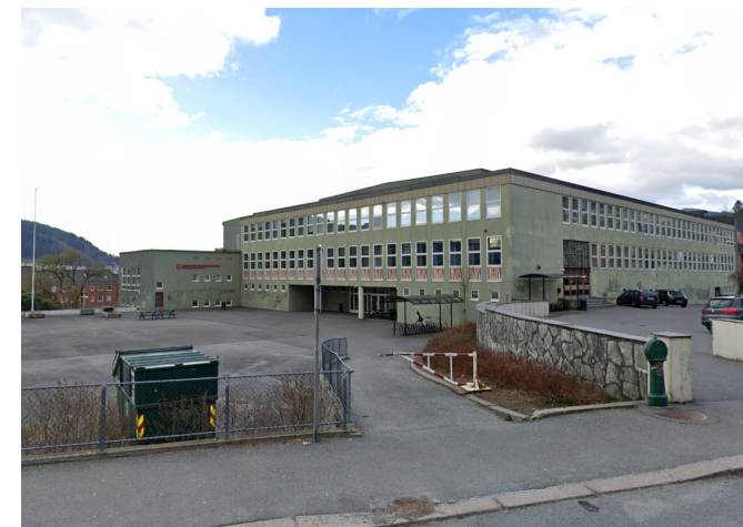
Langhaugen videregående skole (Google street view)
